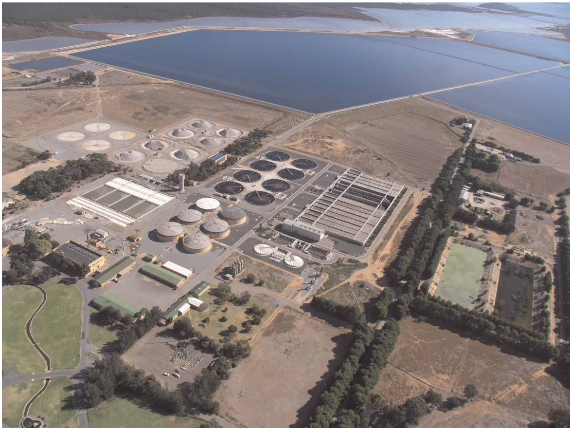
Figure 2 | Aerial photograph of Bolivar WWTP not showing the sludge lagoons, hardstand and stockpiling area.
